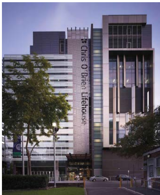
The nine-storey building accommodates cancer surgery, chemotherapy, radiation therapy, complimentary therapy, research and emotional support in the one facility.
