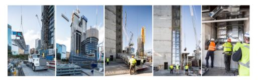
Stemming from an industry-leading A.G. Coombs-Lend Lease initiative, prefabricated services risers are saving hours of on-site installation time and significantly reducing construction risk at Barangaroo.
