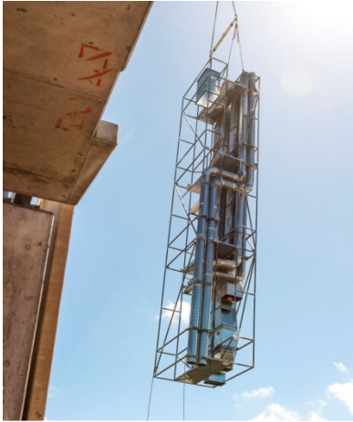
One of the 18 prefabricated riser sections being lifted into position.
