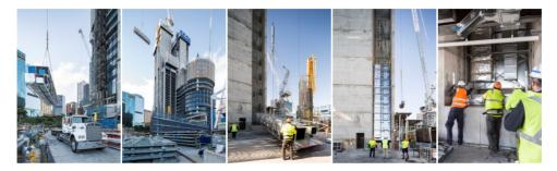
Stemming from an industry-leading A.G. Coombs-Lendlease initiative, prefabricated services risers are saving hours of on-site installation time and significantly reducing construction risk at Barangaroo.
